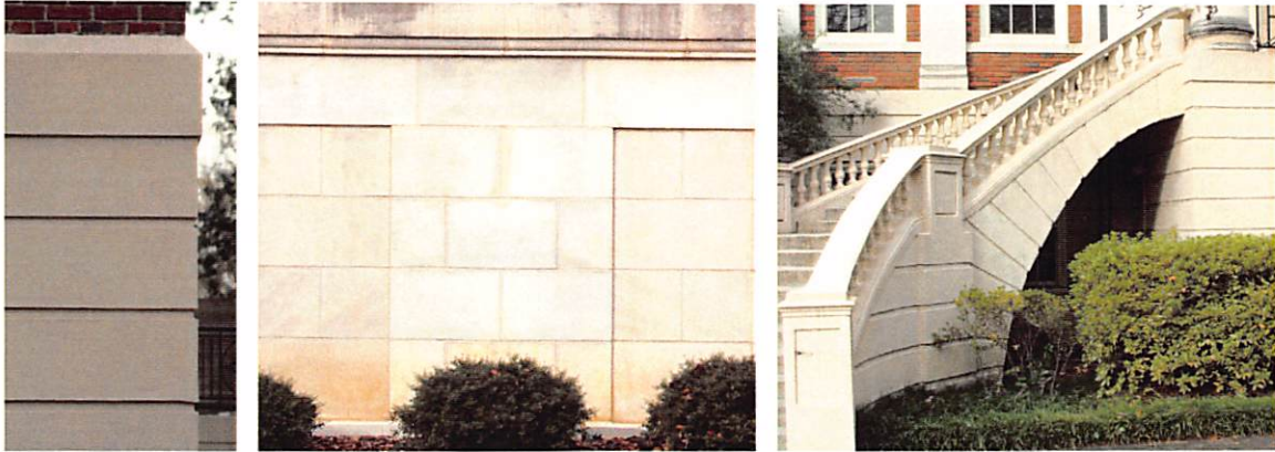
The photographs above show how various campus buildings have used detailing to enhance the massive nature of their bases through exaggerated joints and panel size.
