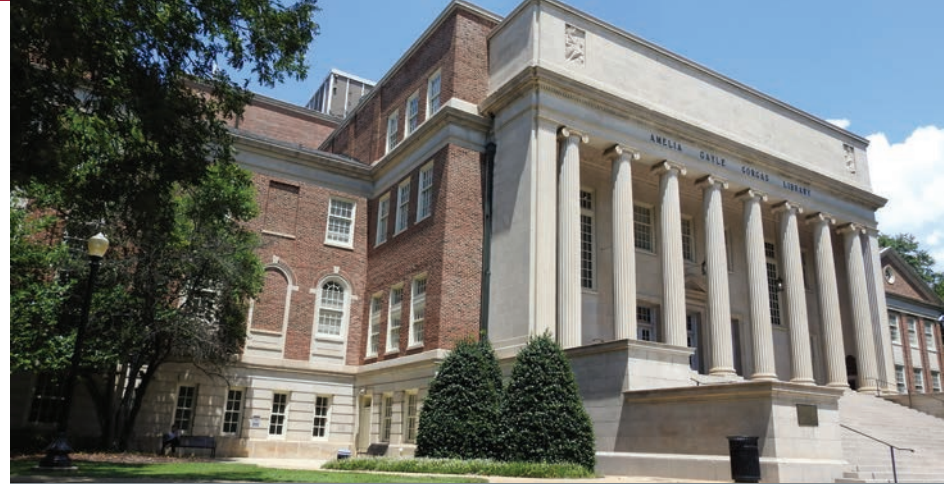
GORGAS LIBRARY RENOVATIONS
