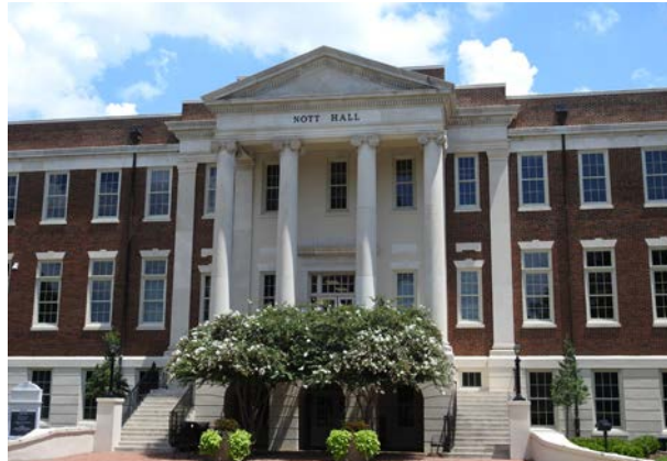
Nott Hall Research Support Facility Fitout
