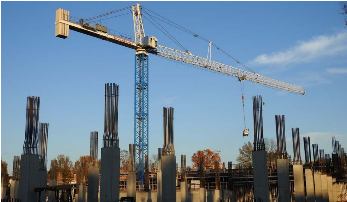
Construction Photo - November 2018
