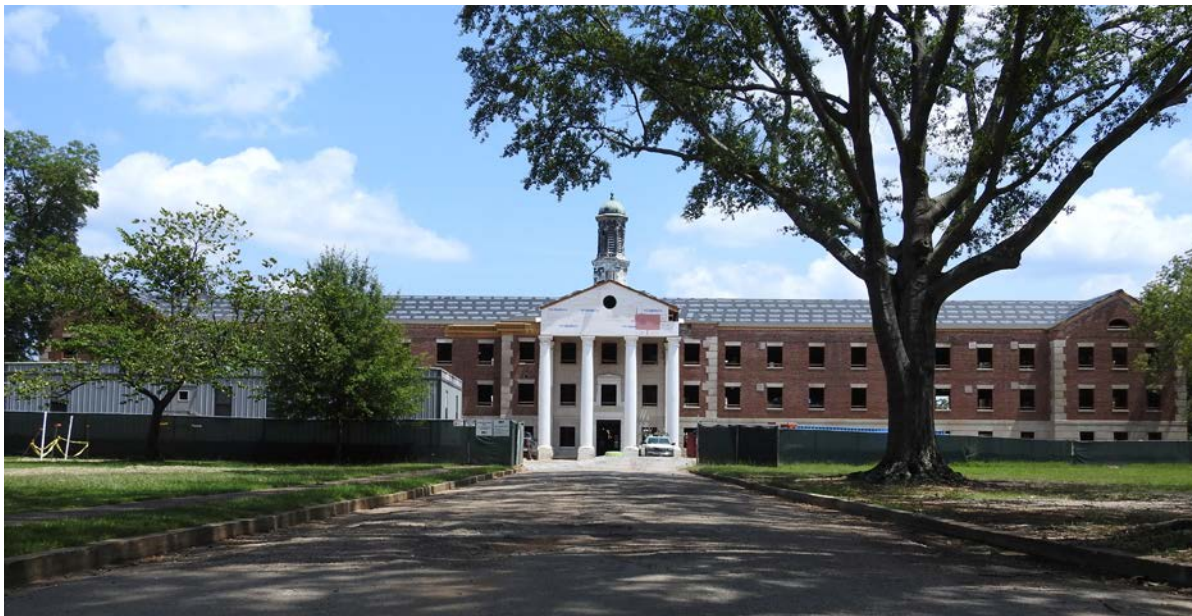
Ongoing renovation at University Hall
