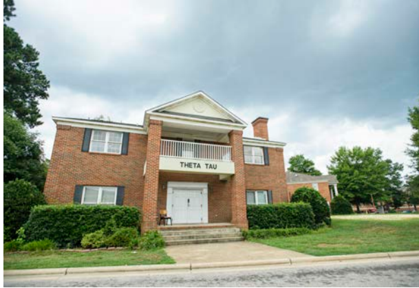
Theta Tau Renovation
