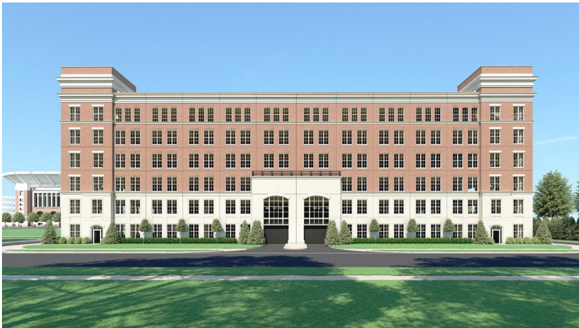
Completed Parking Deck - August 2018
