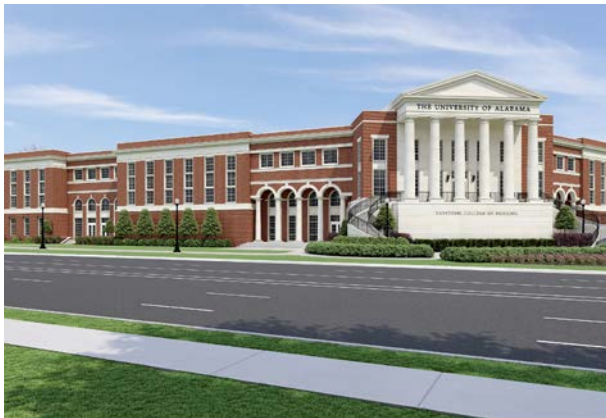
Capstone College of Nursing Addition
