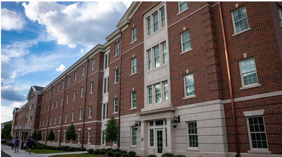
Photo of South Side
