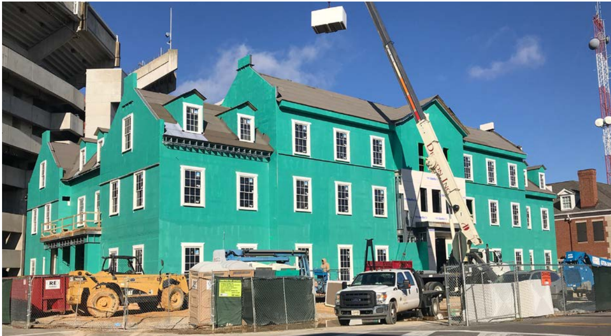
Construction Photo - November 2018
